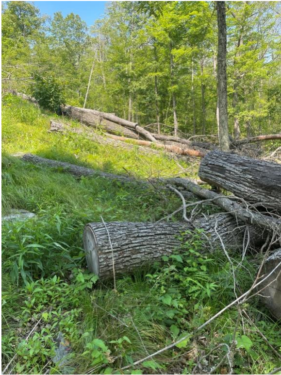
Clearing on steep slopes
